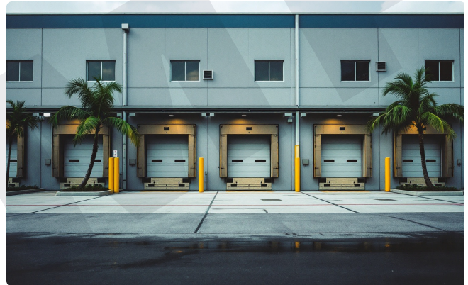
Photo 3. East elevation and dock positions. Tilt-up panels plumb, joints aligned.
